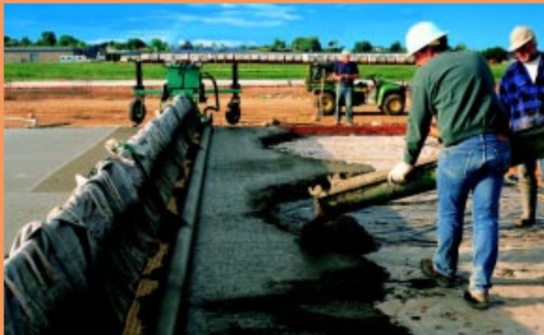
Labor requirements are drastically reduced by the SuperScreed™. Most jobs require a placement crew of only five workers with minimal training.
